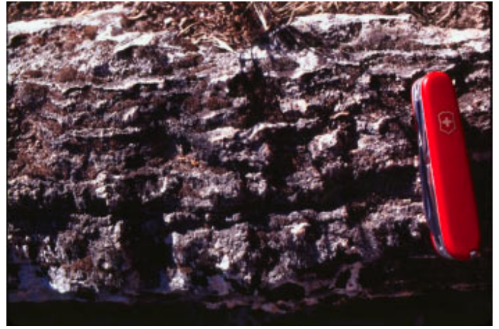
Travertine clogging the aquaduct
